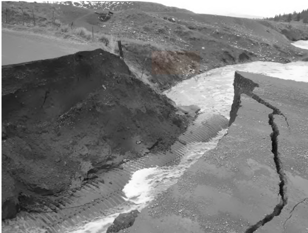
Figure 4-13 April 17, 2010 Flood and Culvert Washout Along Stollsteimer Creek
