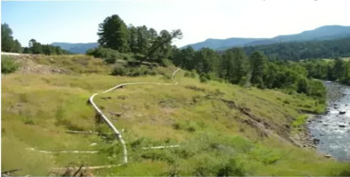
Figure 4-22 Toe of the Jackson Mountain Landslide and Above-Ground Pipeline
